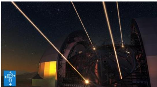
Finally, we have the European Extremely Large Telescope, one of the three extremely large telescopes being built. It will be 39 metres when finished. It is poised to revolutionize astronomy much the same way as Galileo's telescope did a bit more than 400 years ago.
